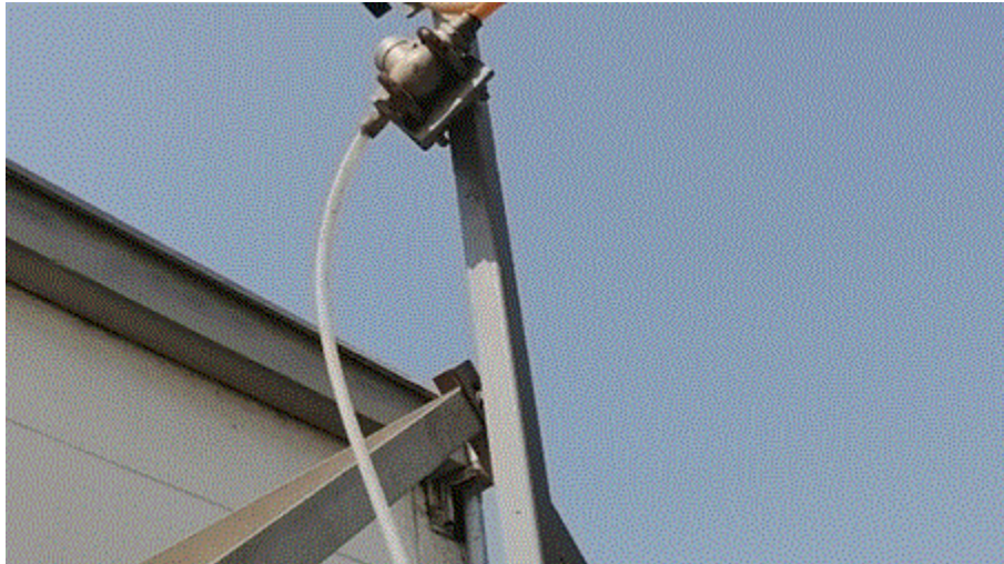
Fig. 8. Check valve
